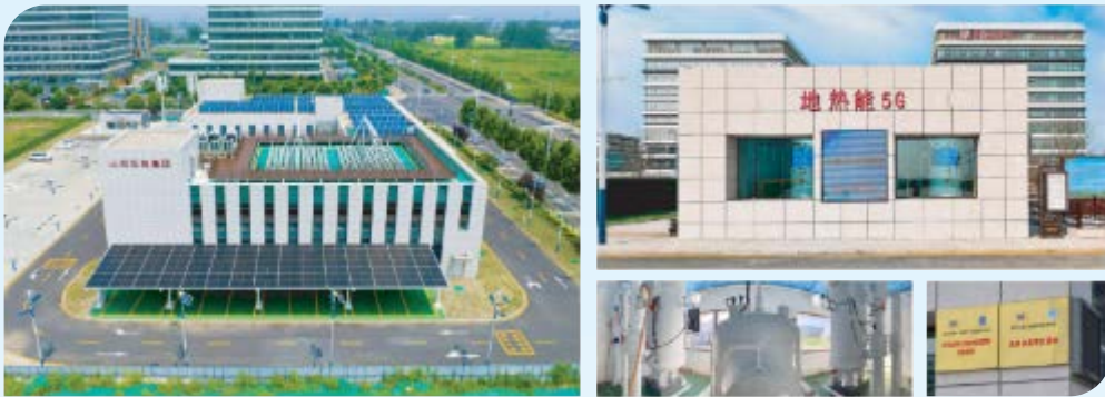
Image of the Energy Island No. 1 Project in Shanxi Transformation and Comprehensive Reform Demonstration Zone
