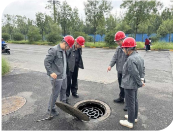
Valve Chamber Inspection
